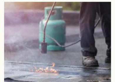
Sheet applied membrane is a type of waterproofing system product offered by Nippon Paint.
