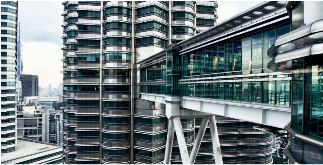
The 750-tonne double-decker skybridge, which is 58.4m long and 170m above ground, acts as the connector between the two towers on Level 41 and 42. Interestingly, the bridge is not fully attached to the main building to give allowance for small movements.
