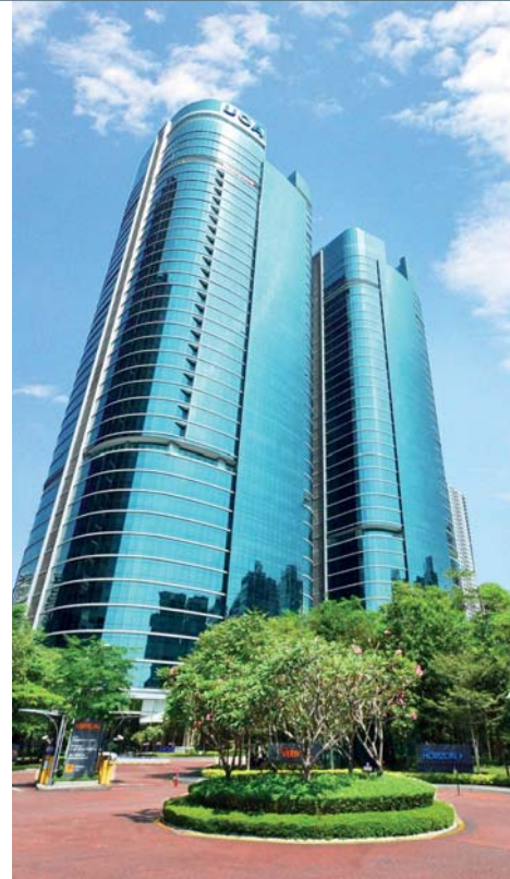
The REIT acquired UOA Corporate Tower, which has a net lettable area of 732,217 sq ft, for RM701.65 million in December 2020
