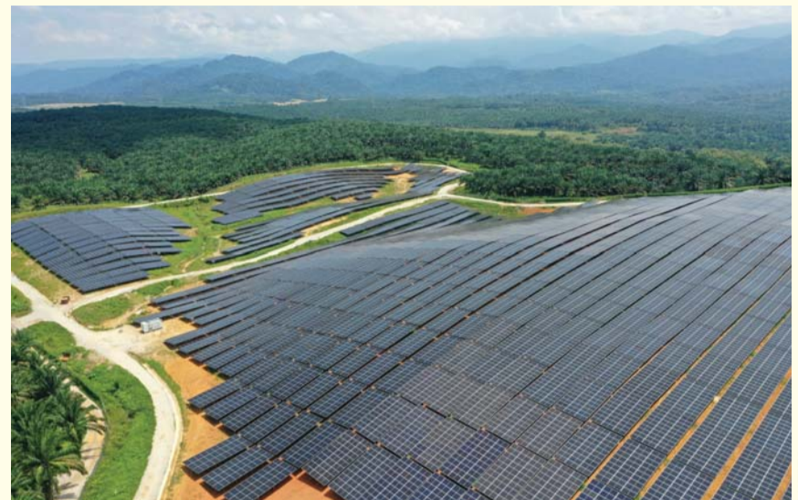
Solar project by Ranhill Utilities
