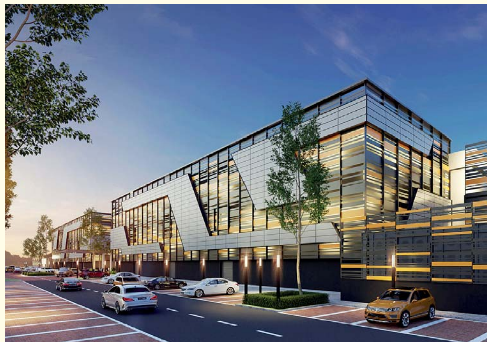
The YTL Green Data Center Park is said to be the first in Malaysia to be co-powered by renewable solar energy on-site
