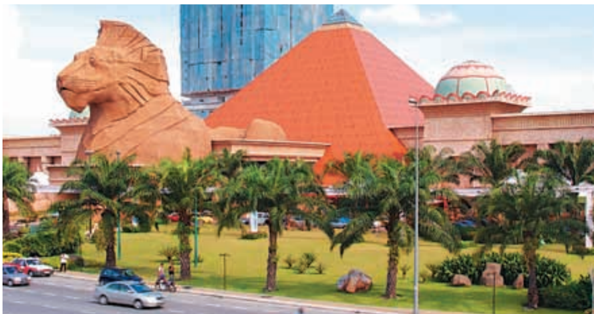
A new wing is being constructed at the Sunway Pyramid Shopping Centre. It will have a state-of-the-art design and facilities and is expected to be opened in April 2007
