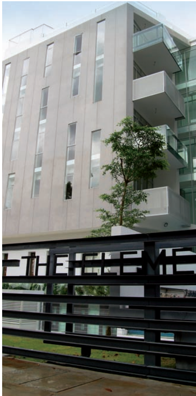
The 17-unit boutique apartment project, The Element at Stevens, along Stevens Road has just received its temporary occupation permit
