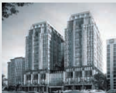
SPPK Building, Damansara Heights
