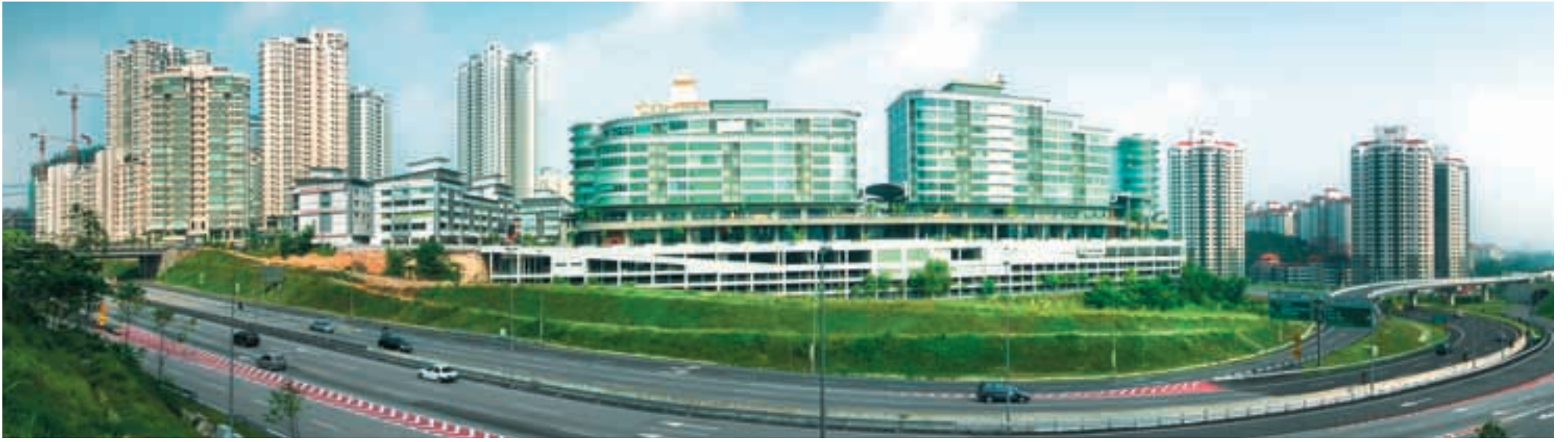
Solaris Mont'Kiara, view from the highway
