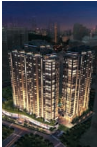
The launch of St Mary Residences Tower C in June 2009 surprised everyone with a take-up rate of 80% within three weeks averaging RM1,000 psf
