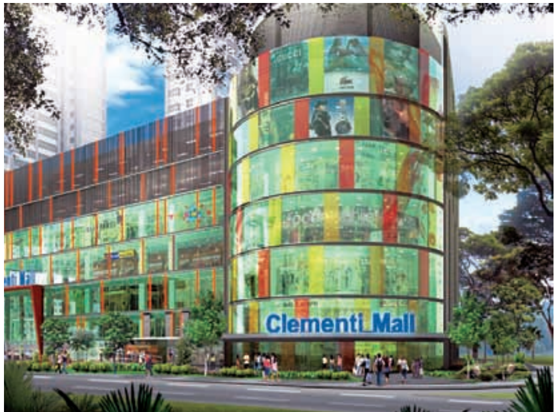
Artist's impression of the Clementi Mall. The buyer of the 7-storey, 99-year leasehold property will have full flexibility to plan the interior theme.
