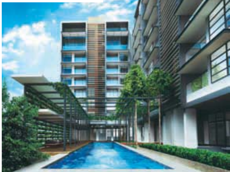
An artist's impression of Seri Ampang Hilir with its hanging gardens and swimming pool
