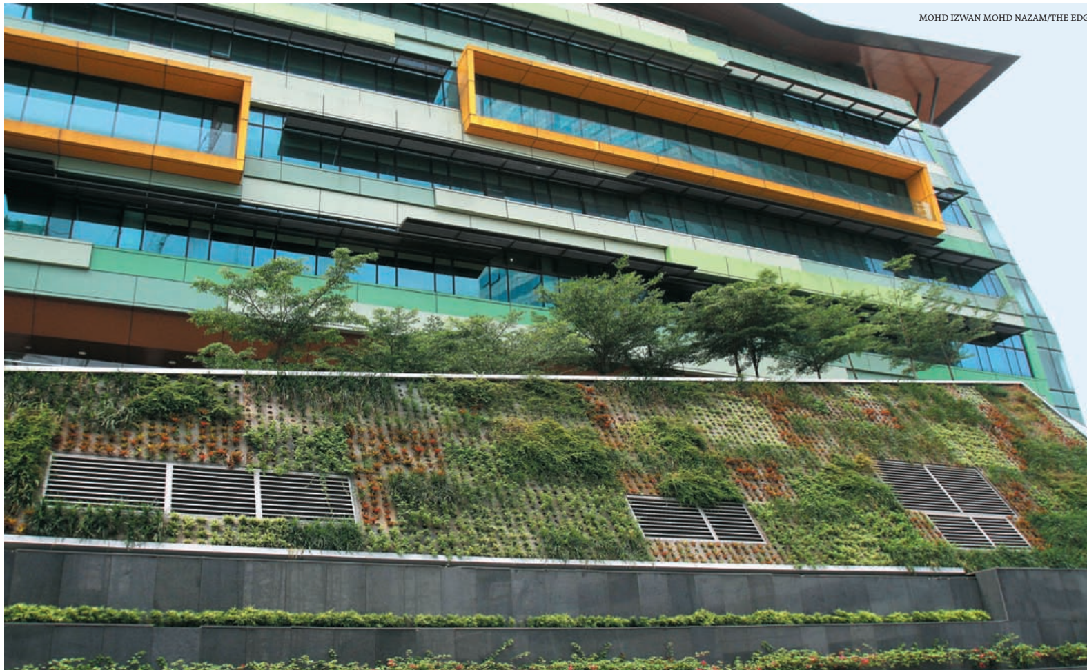
The seven-storey Platinum Sentral boasts not only green and energy-efficient features but also uses the Smart+Connected Real Estate system that cost the developer RM11 million
