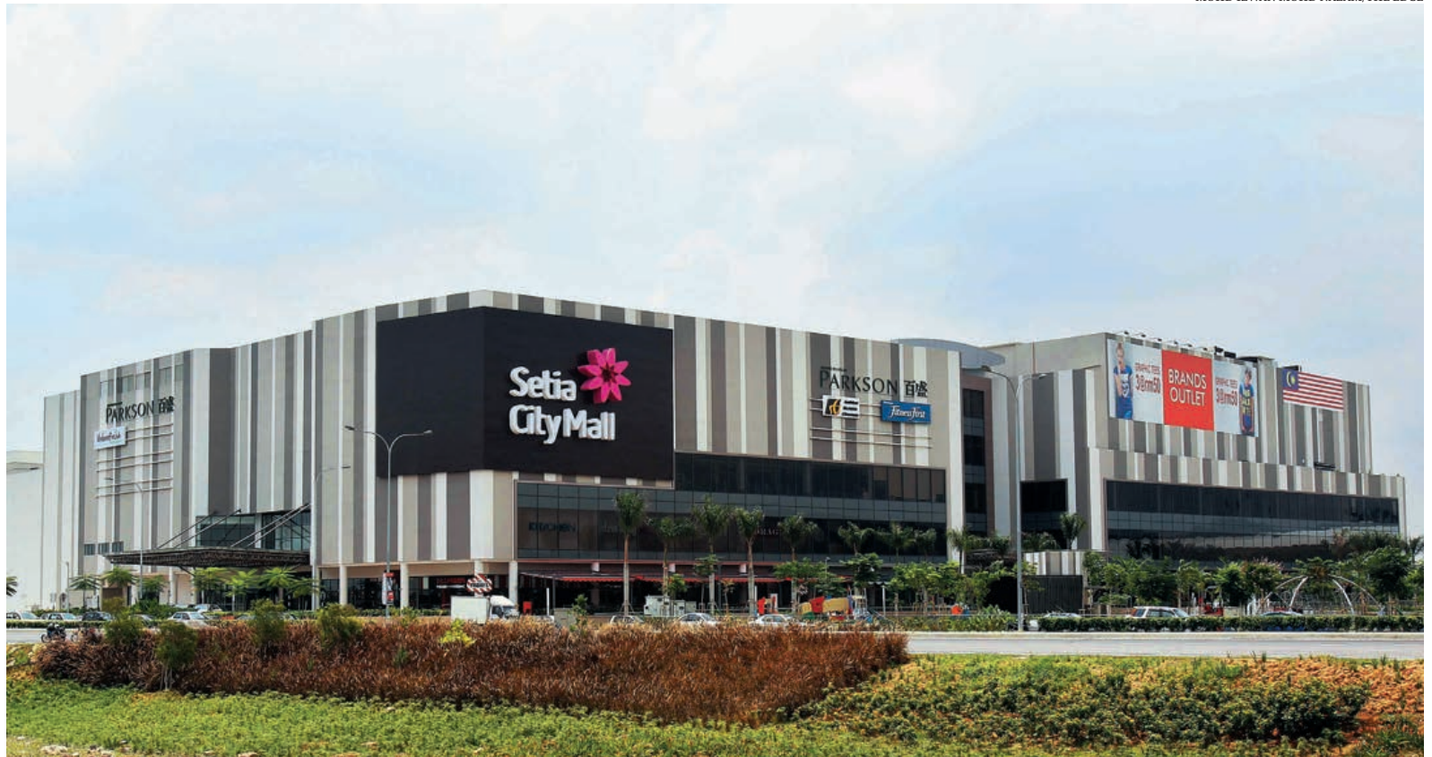
Setia City Mall has an estimated savings of 20% to 30% in energy and more than 40% in water, among others
