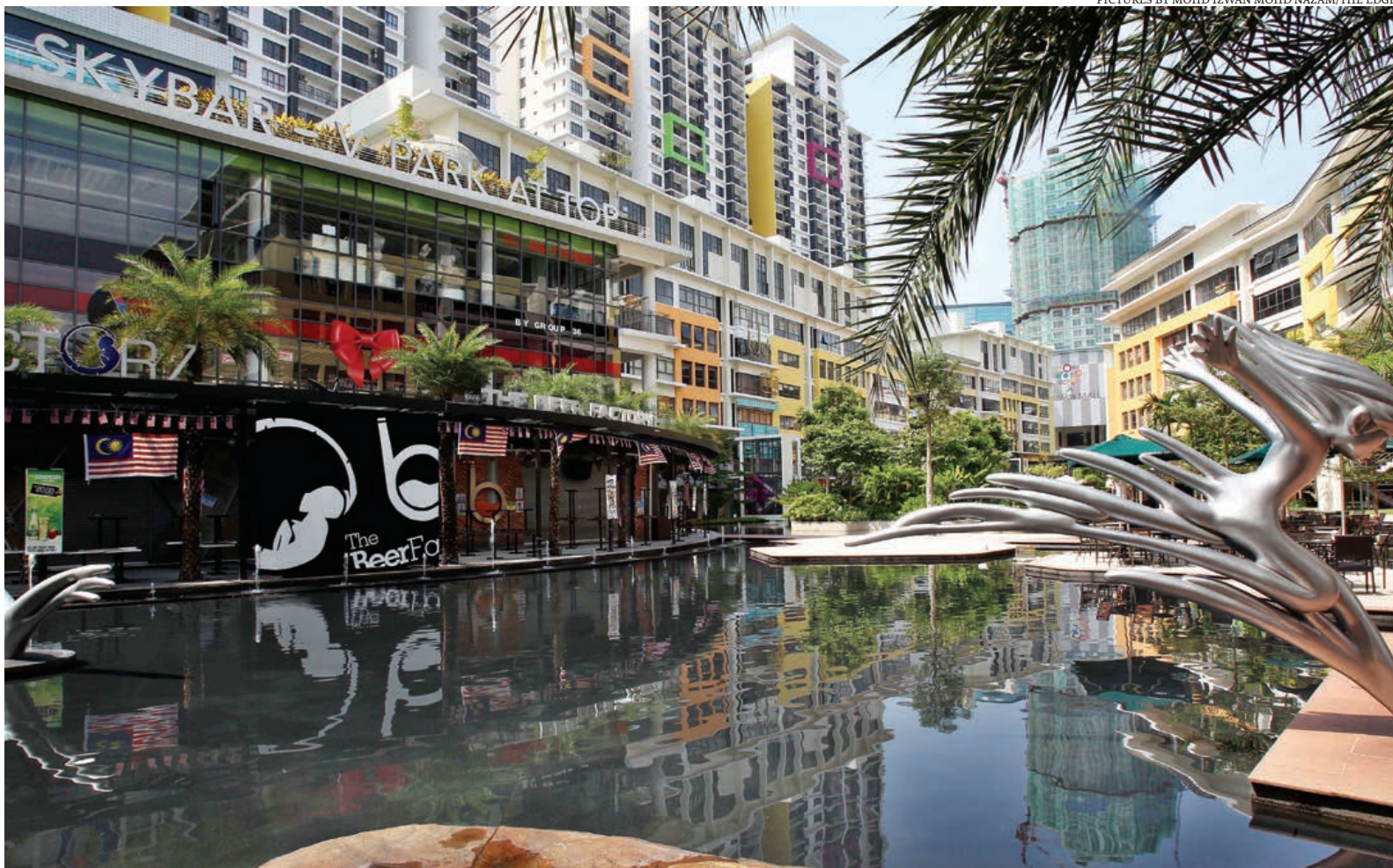
The shopoffices in SetiaWalk has seen capital appreciation of between 12% and 20% per year since its launch in 2008
