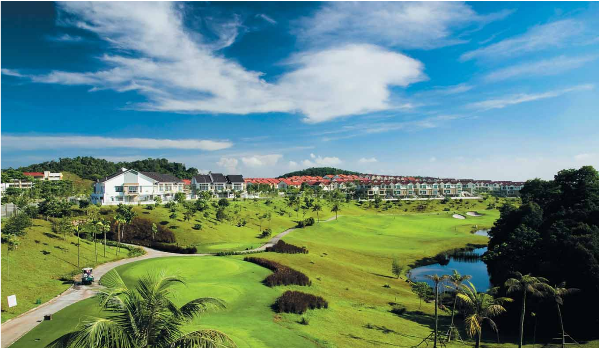
The Golf precinct is enfolded in fairways and greens, where the houses are built in clusters and to match the green environment
