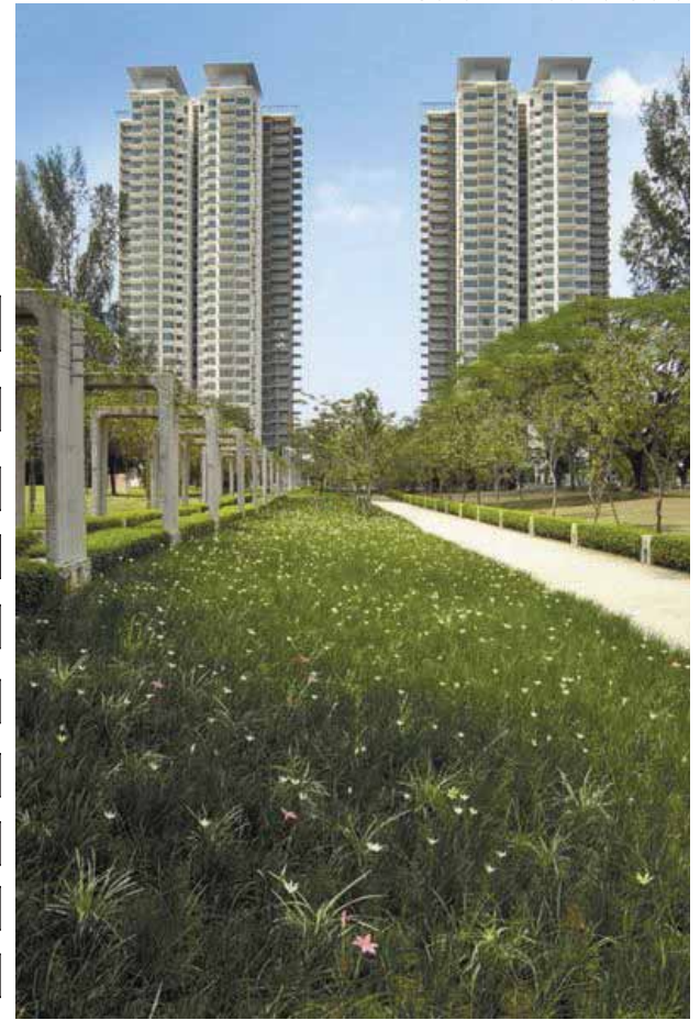
The Maple high-rise in Sentul West
