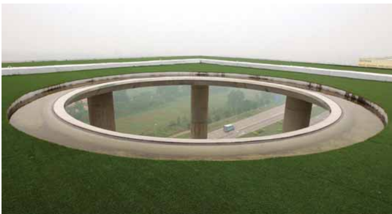
Rainwater is collected at the roof, which goes down to a reservoir
