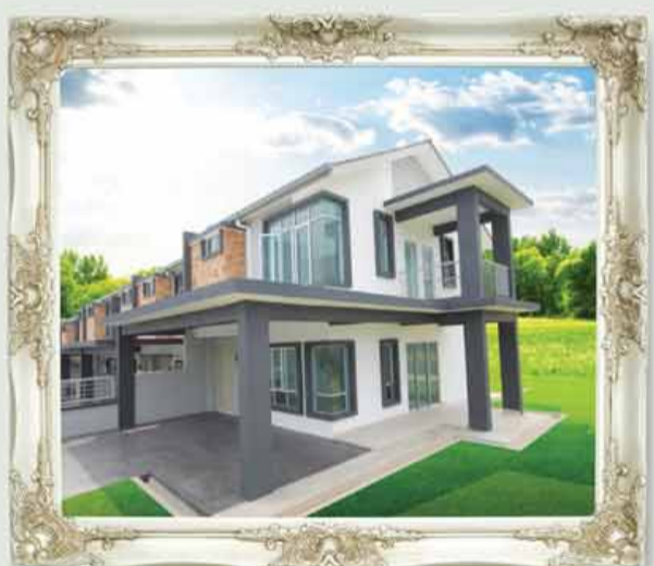
PELANGI SEMENYIH 2 Pelangi Semenyih 2 Completed with CCC Double Storey Terrace Phase 2B • 20'x65' Price From RM500,000*
