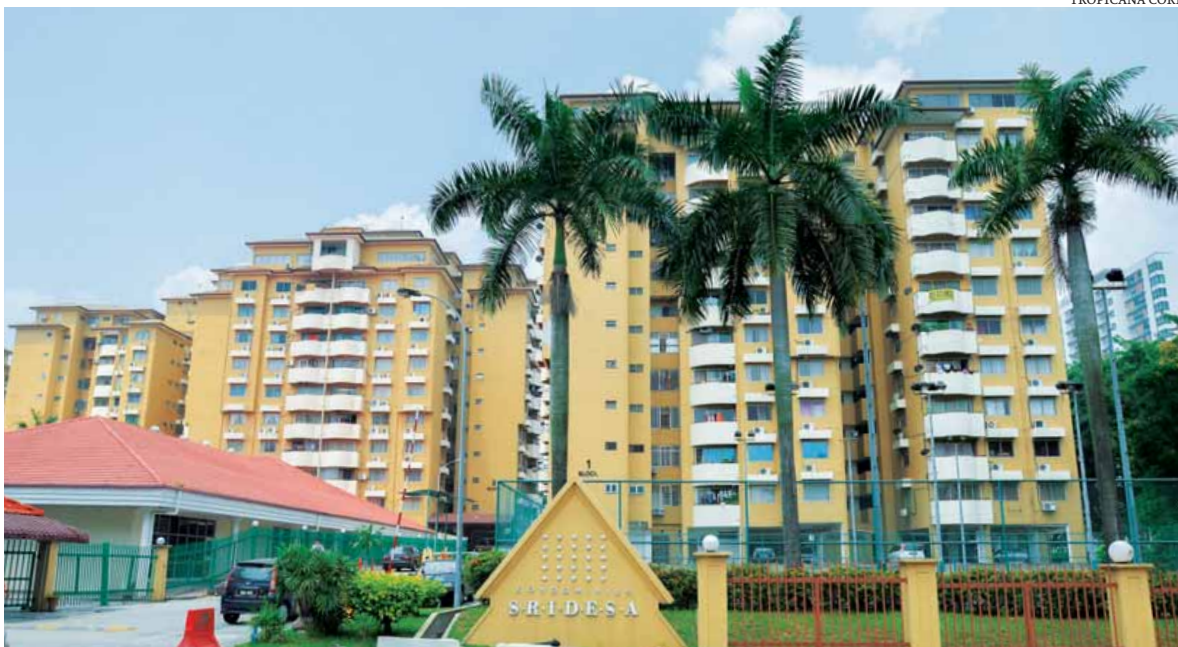
Sri Desa Condominium in OUG, Kuala Lumpur, was developed in the late 1980s
