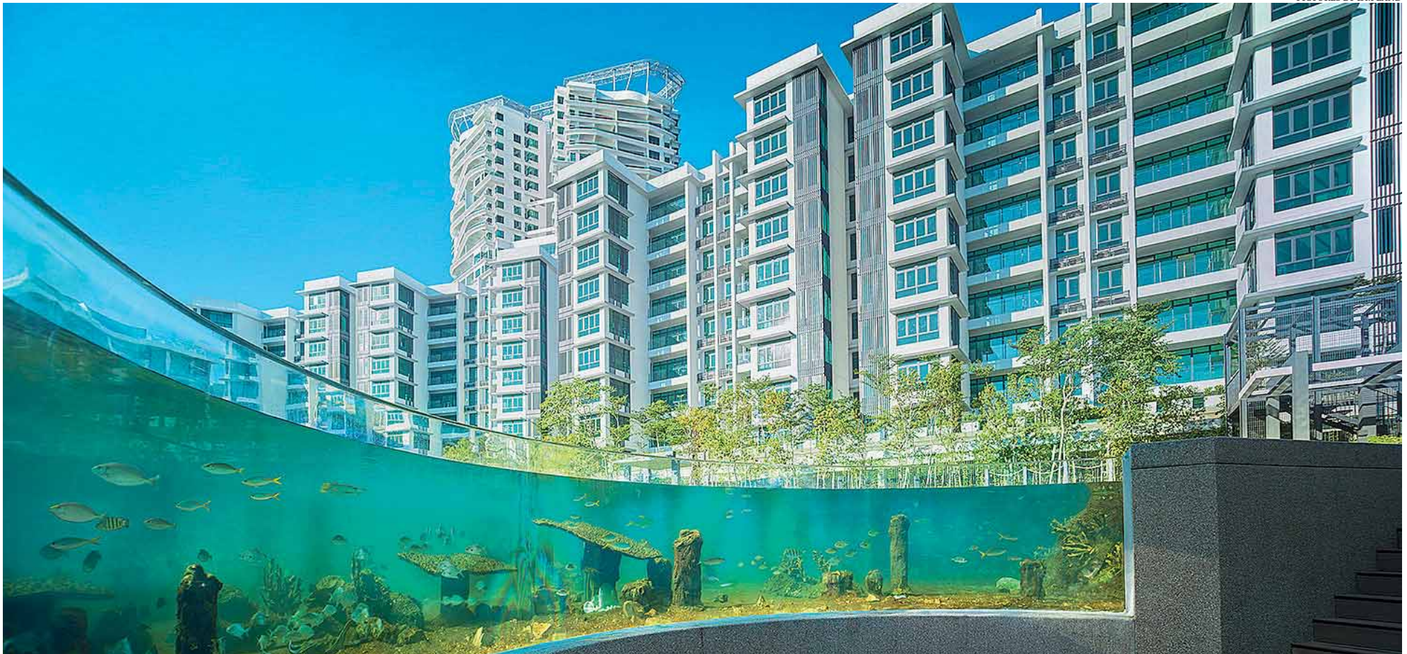
The Waterways has an astonishing six million litres of seawater coursing through channels of glass and concrete
