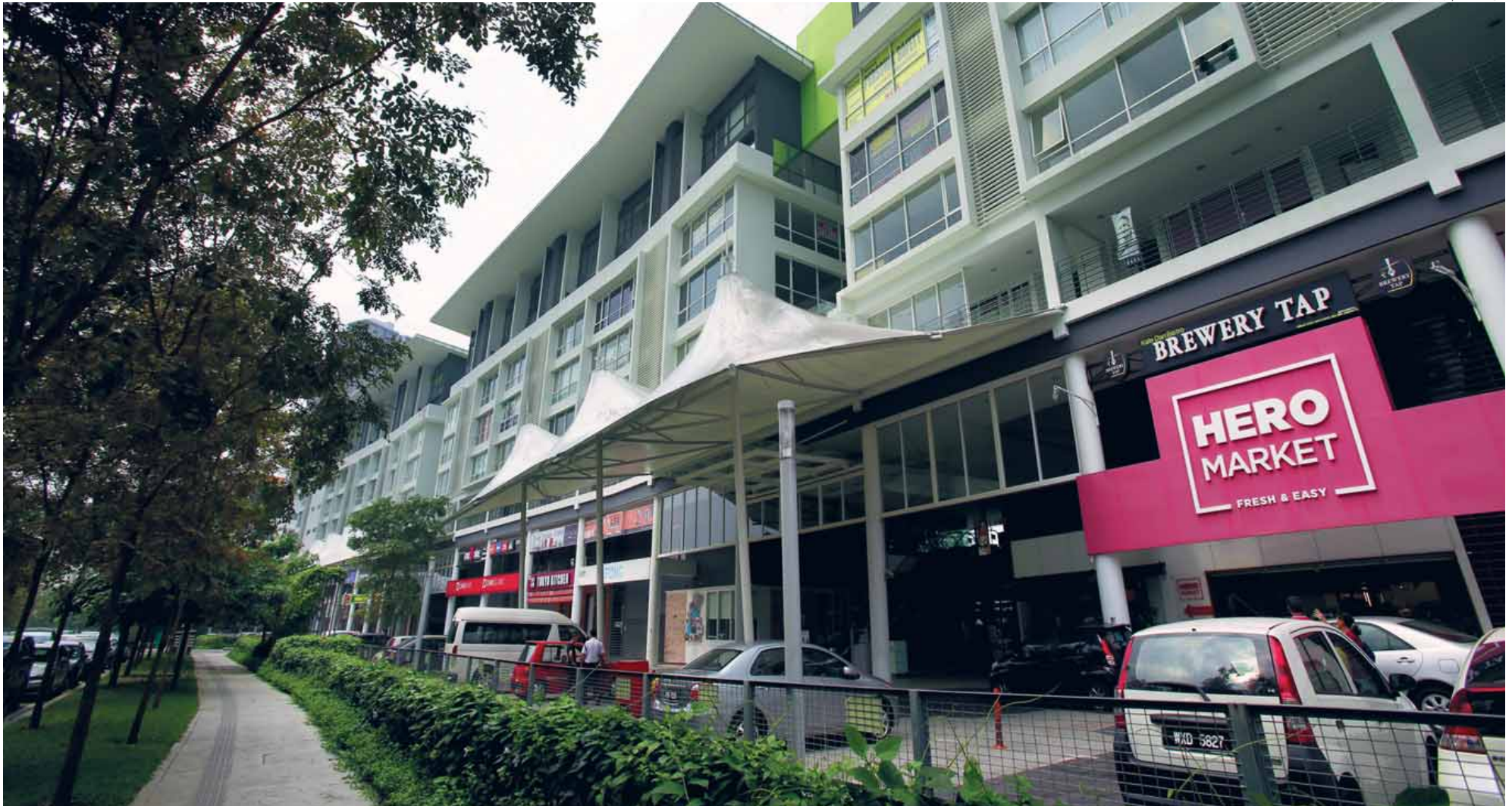
Niche tenants such as Hero Supermarket and Brewery Tap differentiate Ativo Plaza from other retail developments in Bandar Sri Damansara
