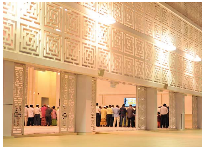
Its exterior features an egg-crate screen that acts as a “skin” to allow maximum natural lighting and ventilation
