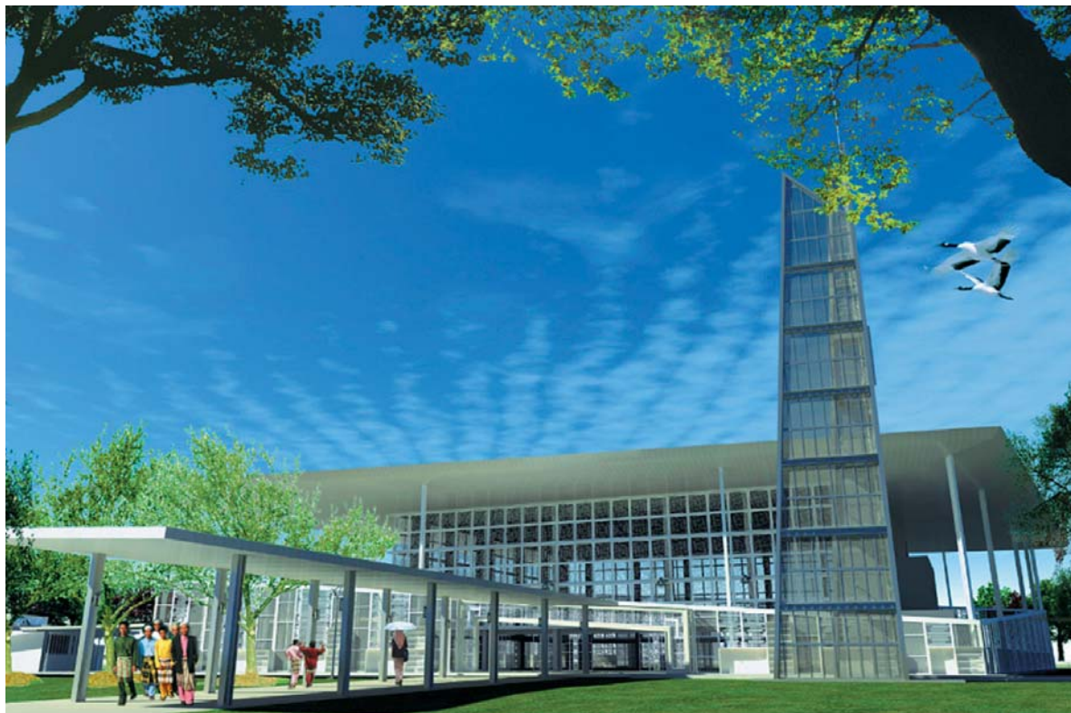
The mosque has an asymmetrical, squarish form that allows good ventilation and sun-path orientation
