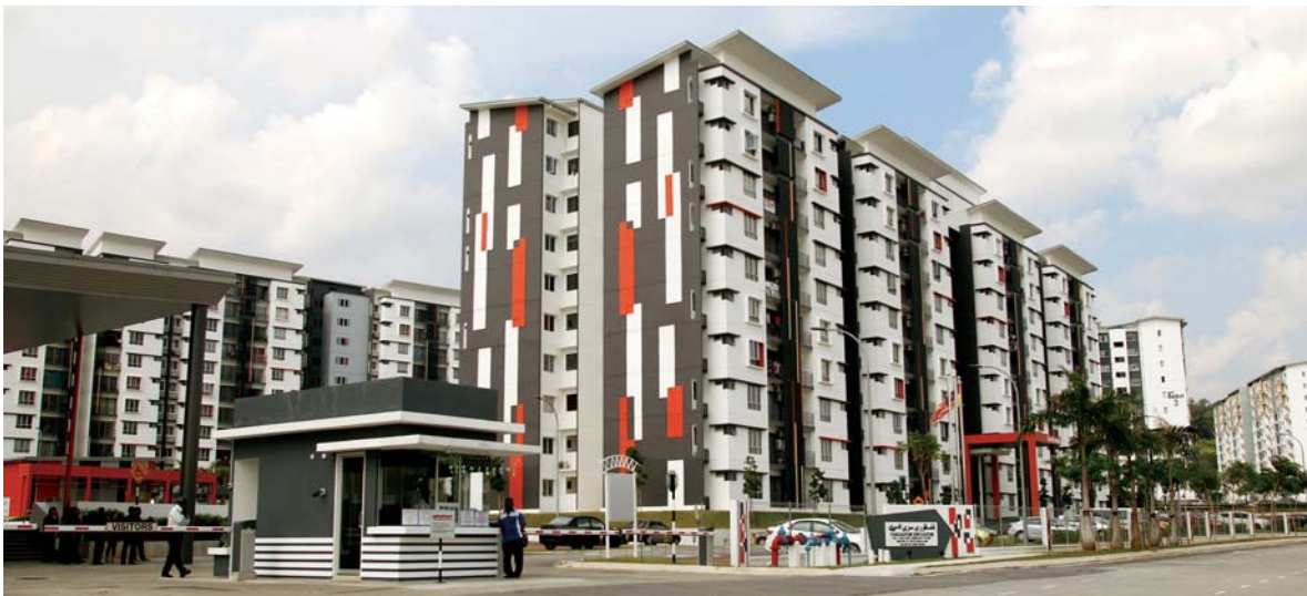
Seri Kasturi's air-conditioned guardhouse against a backdrop of the residential blocks' gable wall murals
