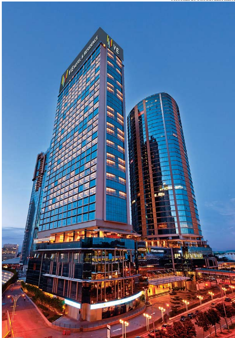
VE Hotel & Residence, which has been open since May
