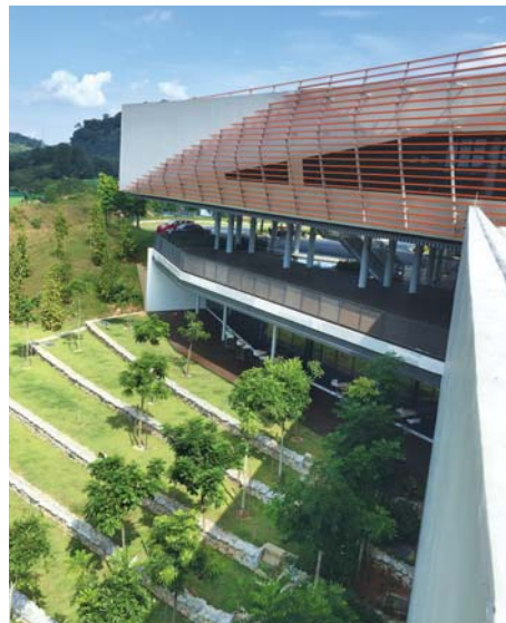
Above: The centre was built in two parts – one is submerged in the terrain, while the second part is cantilevered above it, appearing to float
