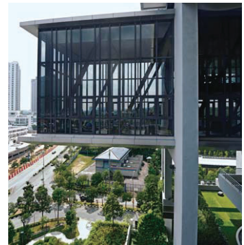
Facilities include a cantilevered gym
