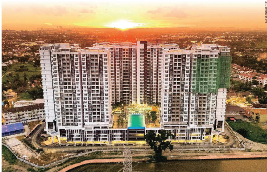
Parkland Residence @ Sungai Melaka had been fully sold by the time vacant possession was delivered, allowing owners to reap the full value of the units
