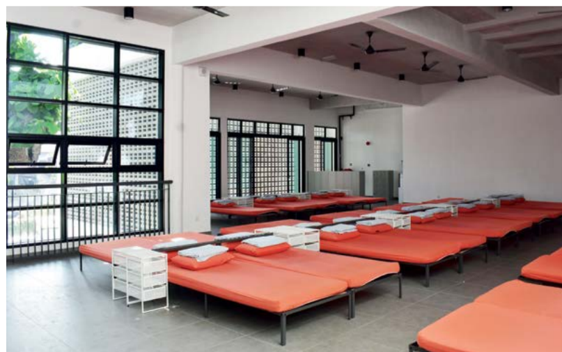
The ventilation blocks in the dormitory walls ensure good air circulation
