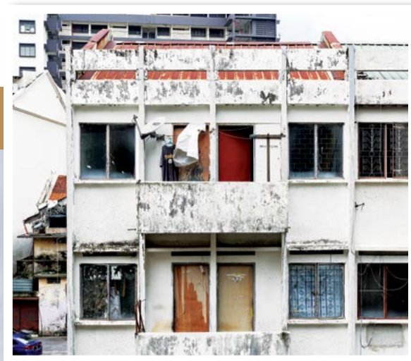
THE ZHONGSHAN BUILDING
