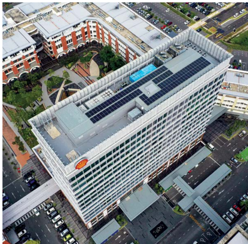
The solar panels on the rooftop of One Shell Square Miri is projected to produce 87,885.79kWh annually
