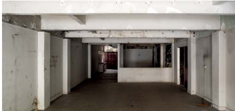
THE ZHONGSHAN BUILDING
