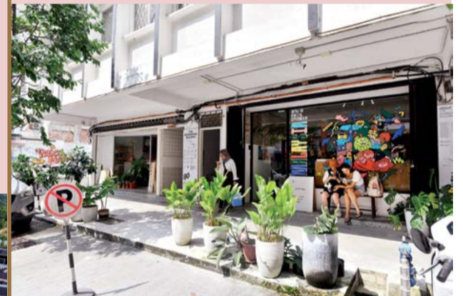
The Zhongshan Building
